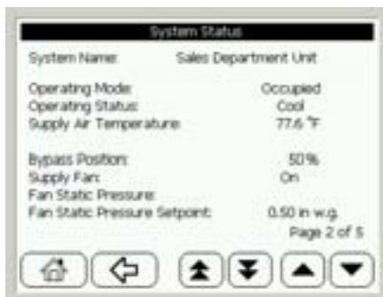
Figure 4. A screen representation from the central control panel illustrating system status
